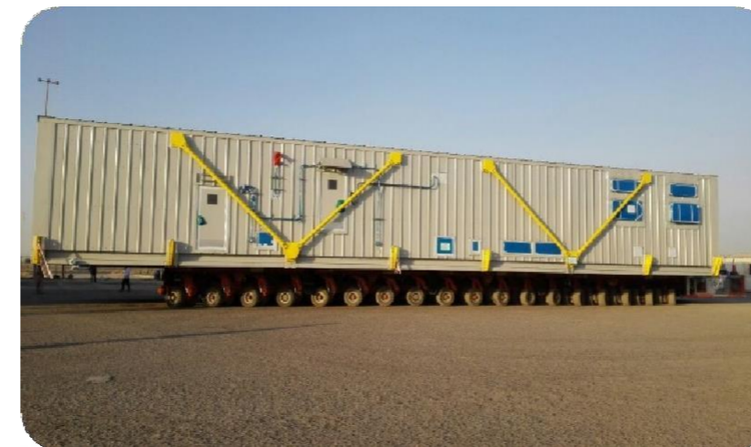
FIELD AUXILIARY ROOM (FAR) Dim: 30.15 * 11.47 * 5.0M (LWH) GWT: 196.10 tons
